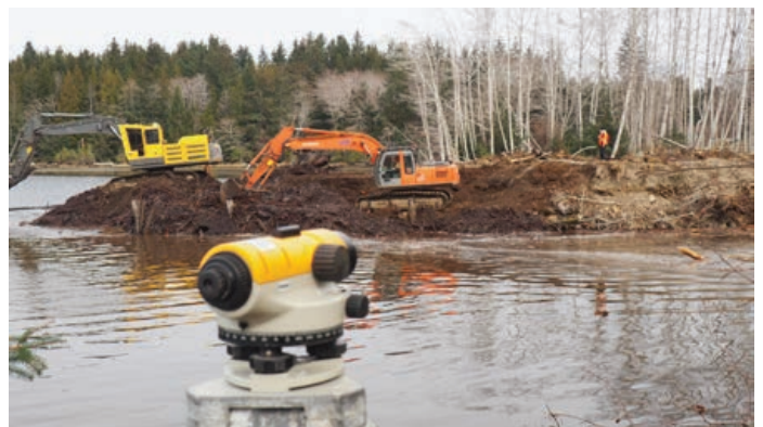
Getting elevations and reprofiling the shoreline. | Photo credit: Peter Dymant
