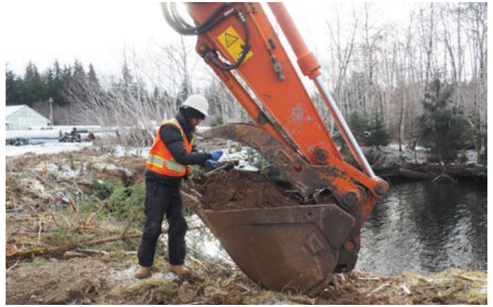
In order to restore T’aanuu eelgrass meadow habitat, tons of infill, which were dumped in the ocean during log sort operations need to be excavated. | Photo credit: Peter Dymant
